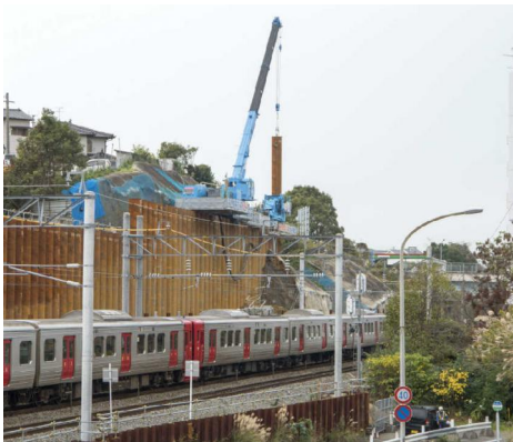
Pile Installation in Progress
