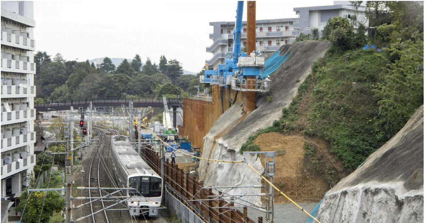
Construction adjacent to train operation
