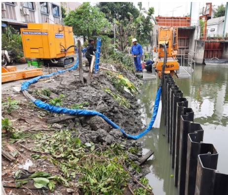
Steel sheet pile revetment
