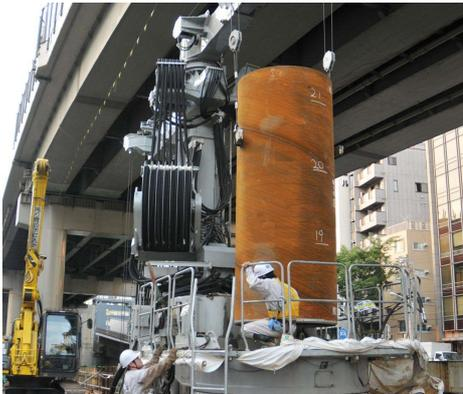
Pitching the Pile by the Hoisting Apparatus
