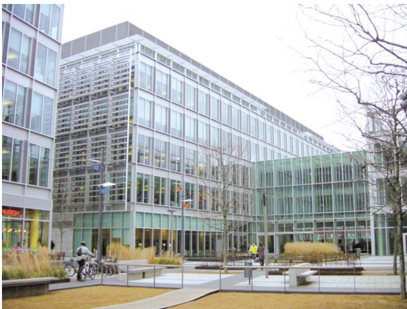
Above Ground, Post Construction - New Building
