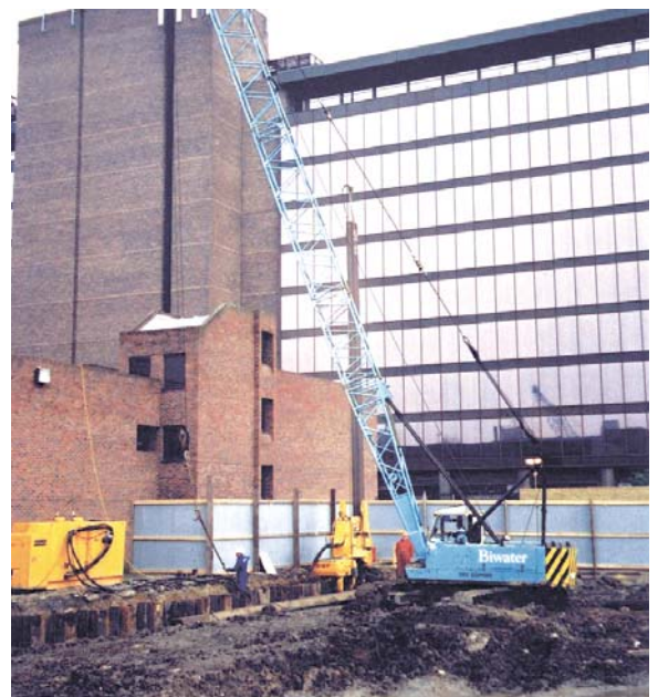
Press-in Work in Progress
