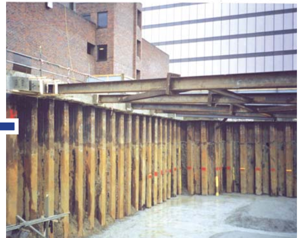
Capping Beam Formed & Excavated
