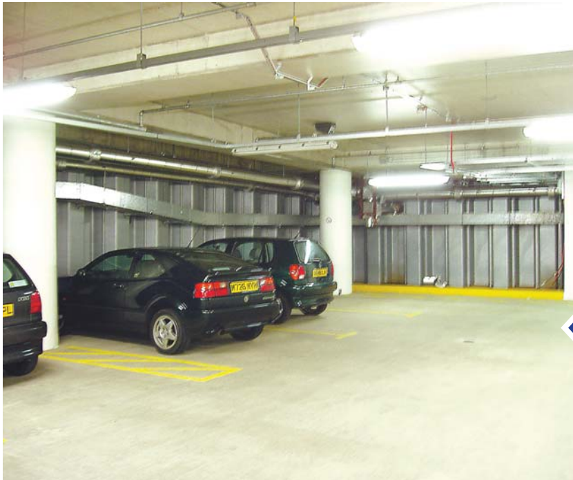
Below Ground, Post Construction - Basement Car Park
