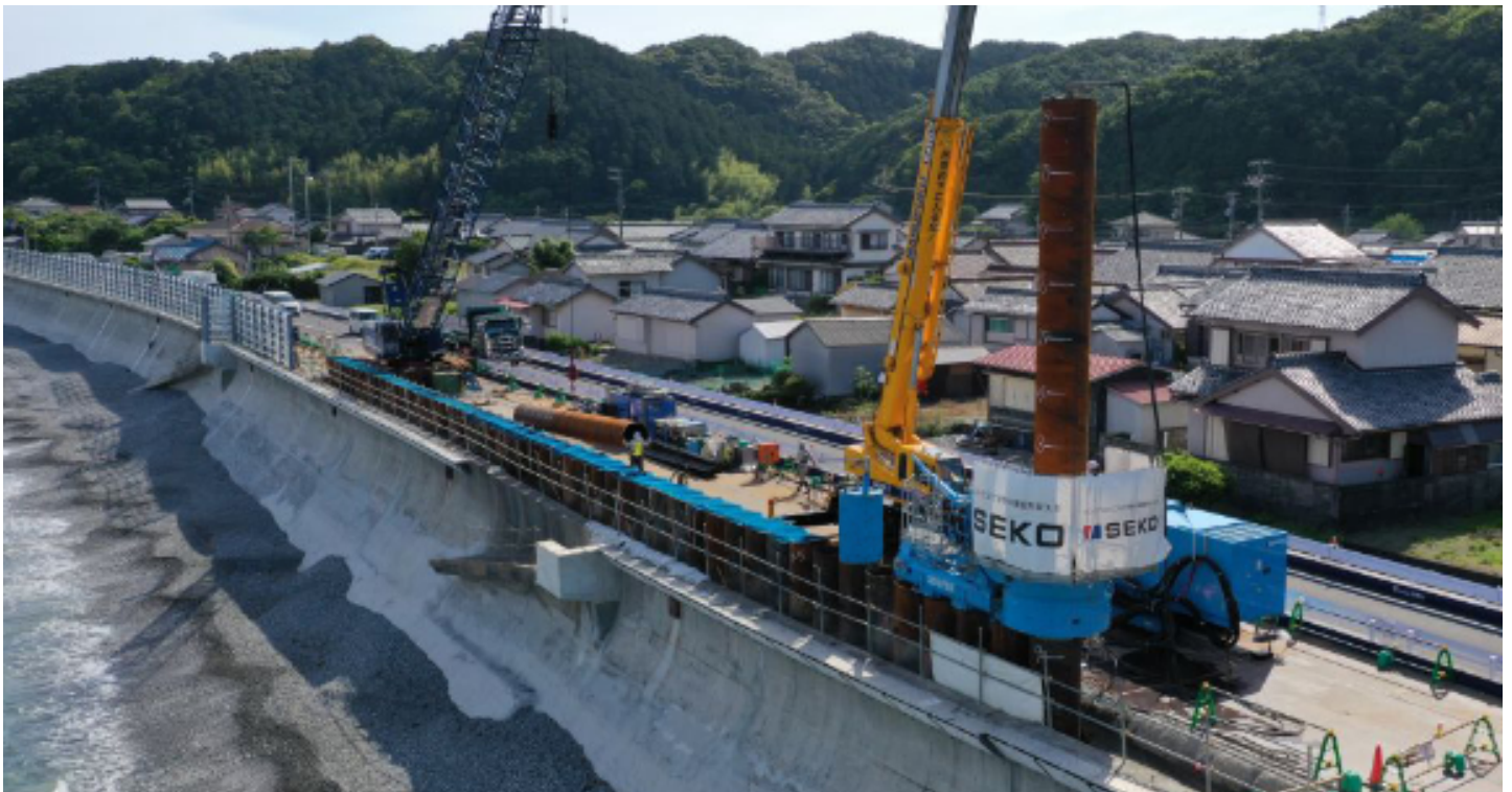
Construction in progress
