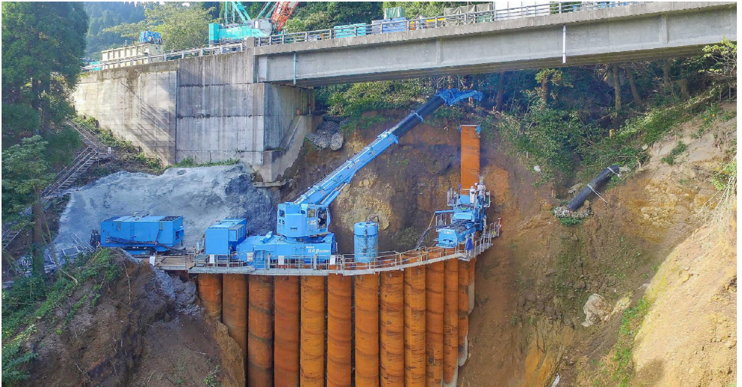
Pile Installation in Progress
