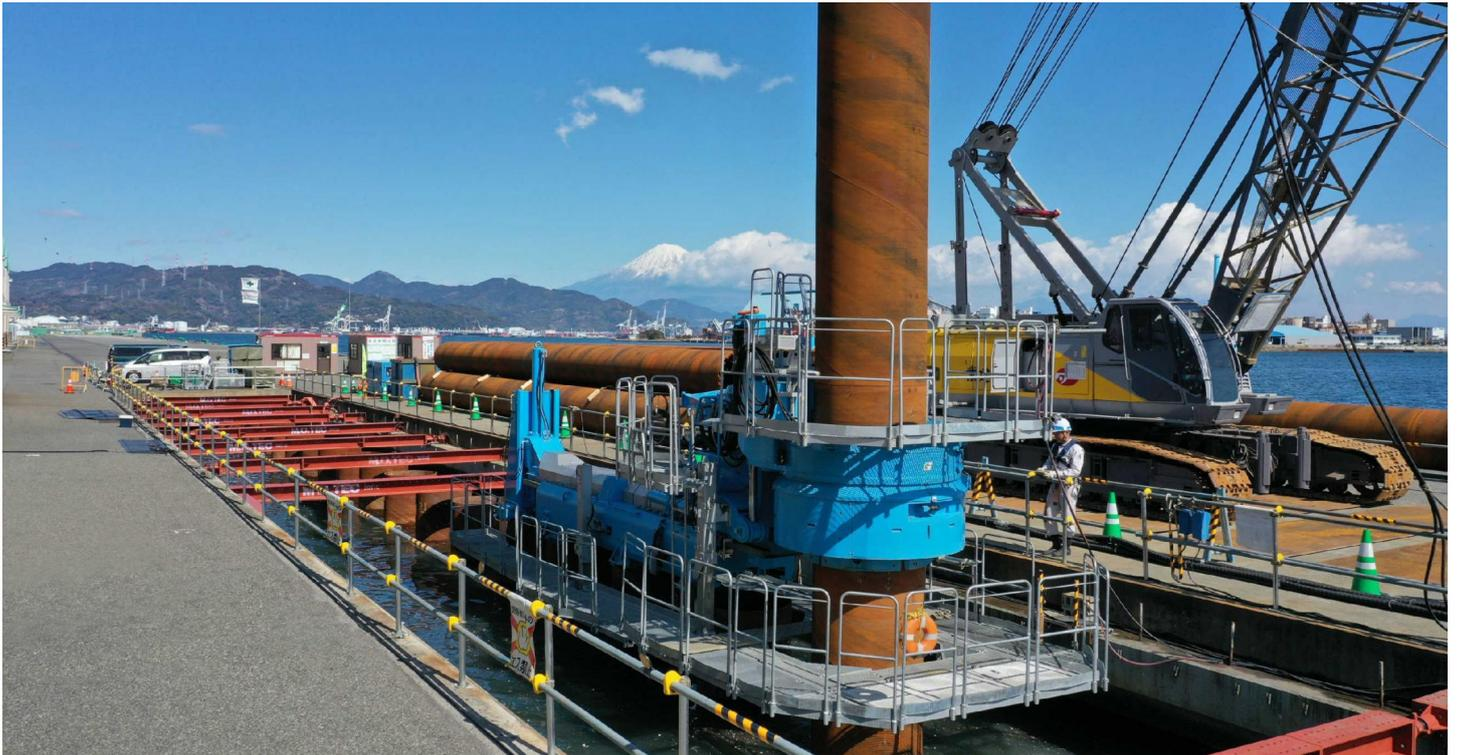
Installing steel tubular piles with skip lock method (F401).
