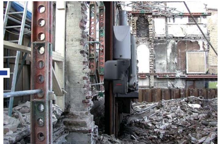
Press-in Work in Progress
