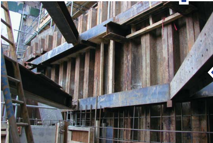
Temporary Frame Works Formed and Excavated
