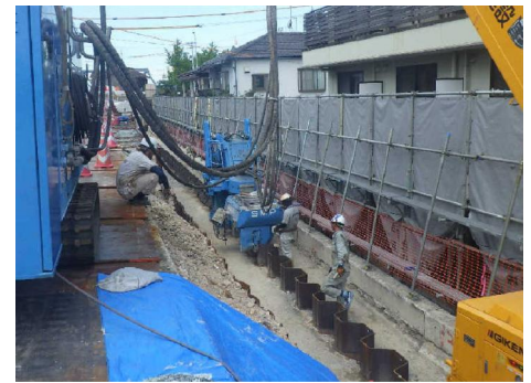
Construction work in progress
