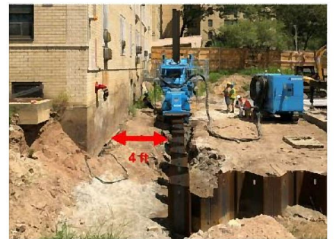
Piling Adjacent to Existing Structure
