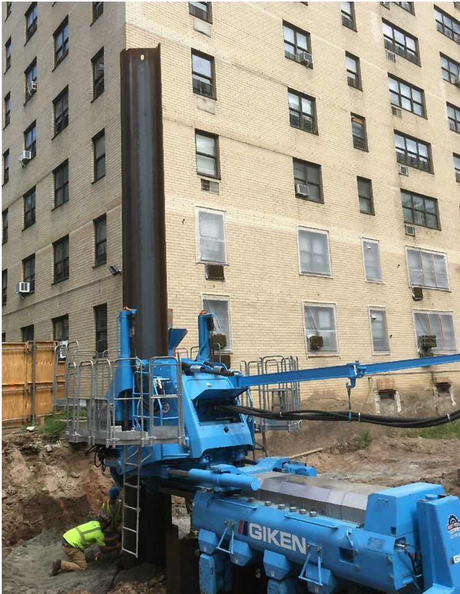
Piling Work in Progress
