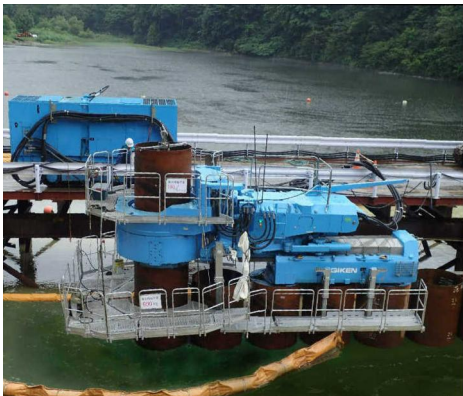
Press-in method in progress
