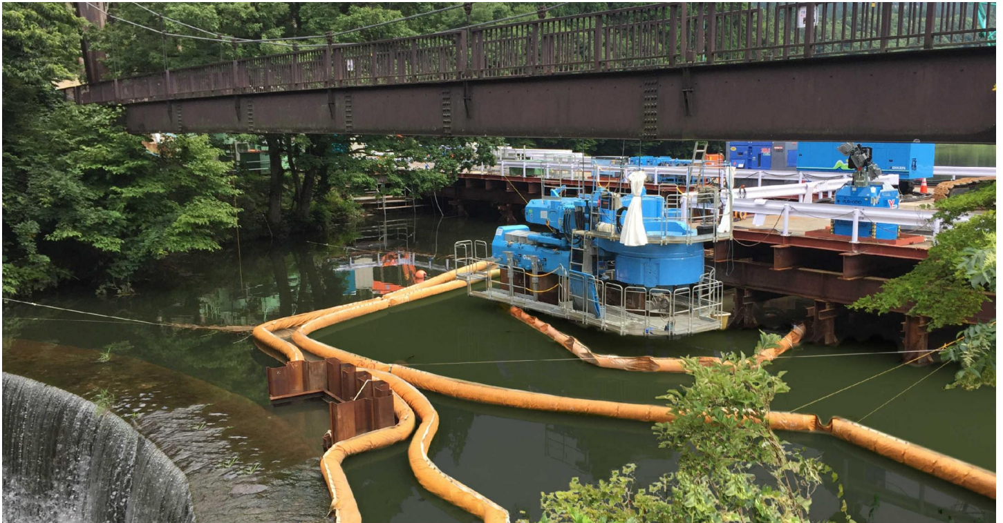
Press-in machine and sand control dam (lower left)
