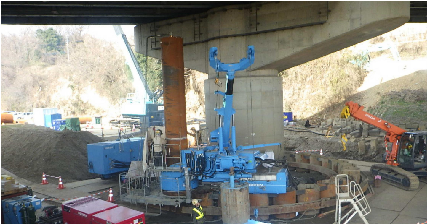
Welding steel tubular piles under bridge
