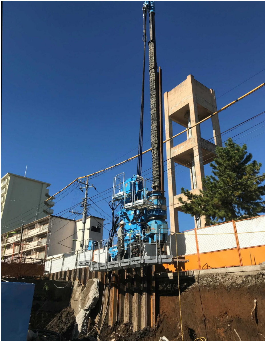
Construction in progress
