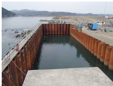
Completion of Pile Installation
